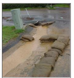
Poorly maintained BMPs can result in significant quantities of sediment being discharged to storm drains.
